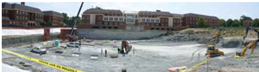
Figure 9: Looking south during first elevated slab construction. Photo by THP.
